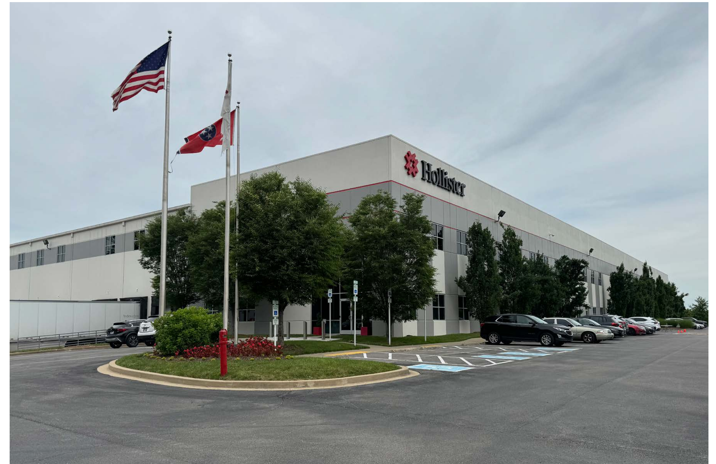
Distribution center in Mt. Juliet, Tennessee
